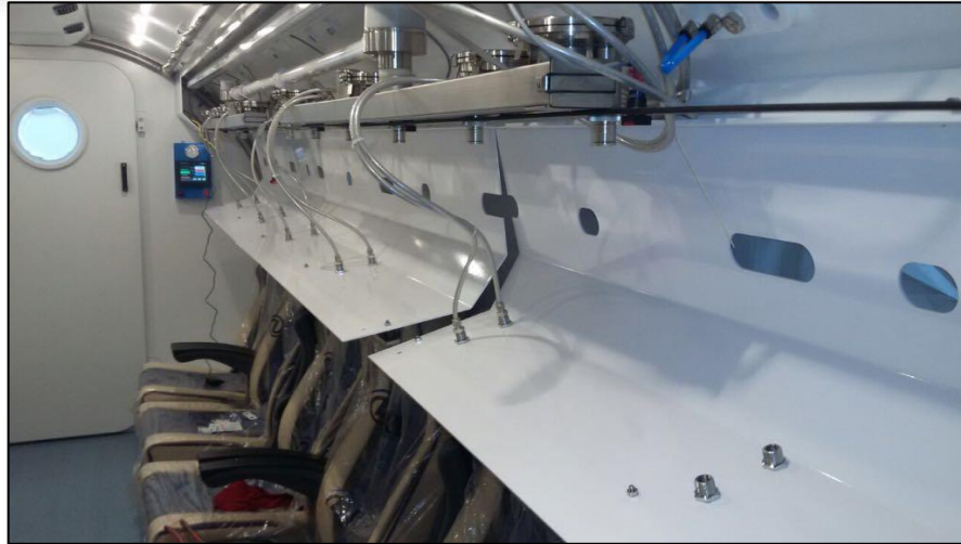
Figure 7 - Oxygen BIBS System
