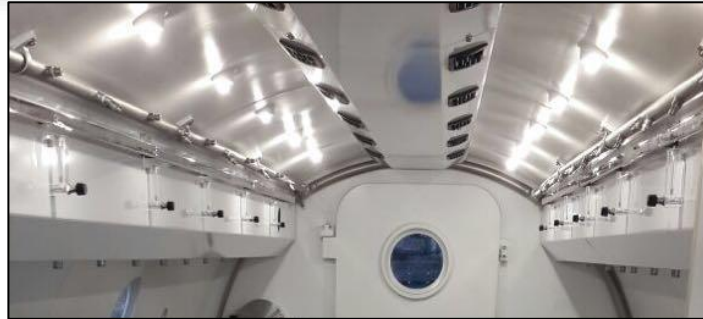
Figure 9 - OKSEA-LUX Cold-lights (inside view)
